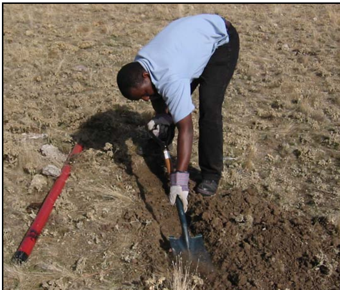
Fig. 2-44: Digging a shallow trench for a coil sensor.
